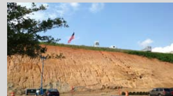
Future plans for the 1,400-acre Tryon Resort include a hotel that will be built by Salamander Hotels & Resorts. The hotel is planned to have an entrance with two stories above ground on top of a ridge, while the backside will be built into the ridge itself, shown here, overlooking the Tryon International Equestrian Center. (Kristen M. Clark / The Palm Beach Post)
