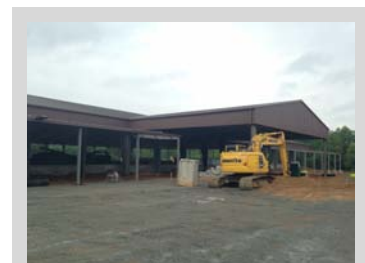
The covered arena at the Tryon International Equestrian Center, shown here under construction in early June, is 400 feet long by 240
